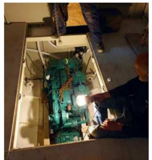
ABOVE: Safely installed and ready to go with a wing engine as a back-up
