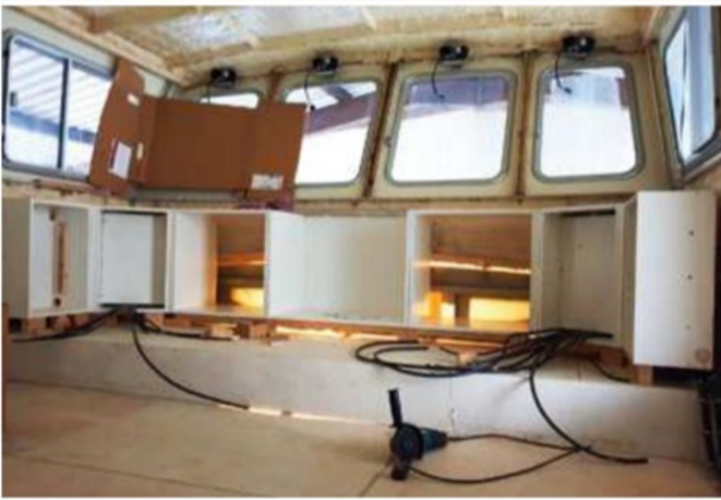
ABOVE AND RIGHT: After painting and insulating, work on fitting out the interior could begin in earnest
